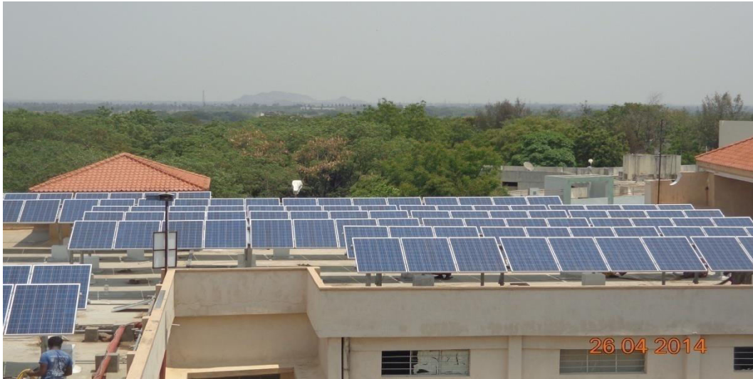
Fig- Roof Top Solar Energy Generation system
